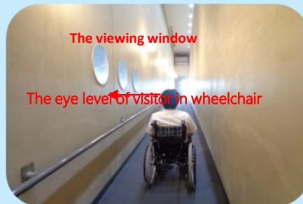
A barrier-free route where a person in a wheelchair won't be able to see the display through the window as they pass by.
