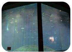
Cloudy acrylic panels and deterioration of glued parts
