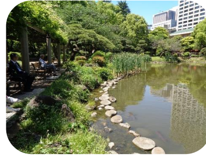
<Kumogata Pond’s revetment>
